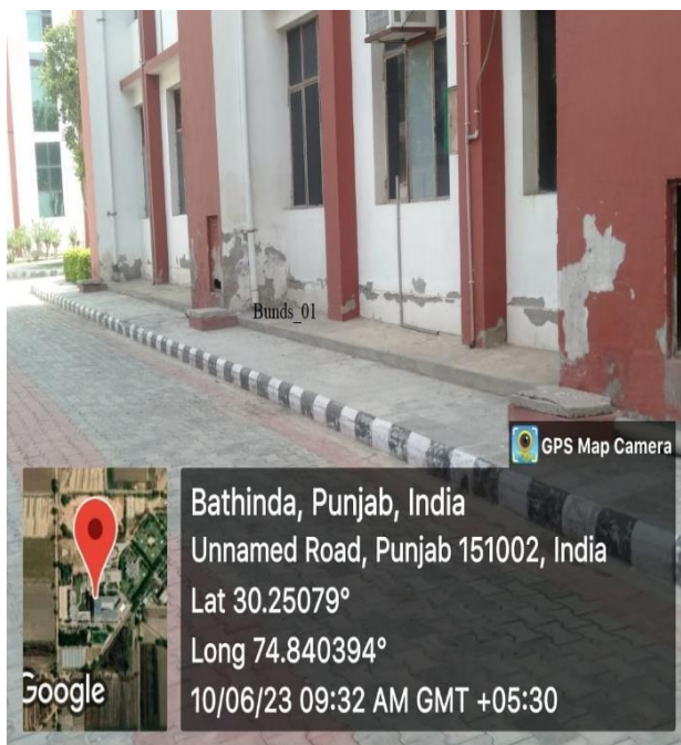
Figure 9: Water conservation (Bunds)
