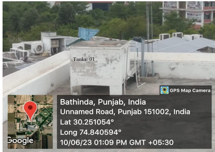
Figure 8: Water conservation (Storage Tank)
