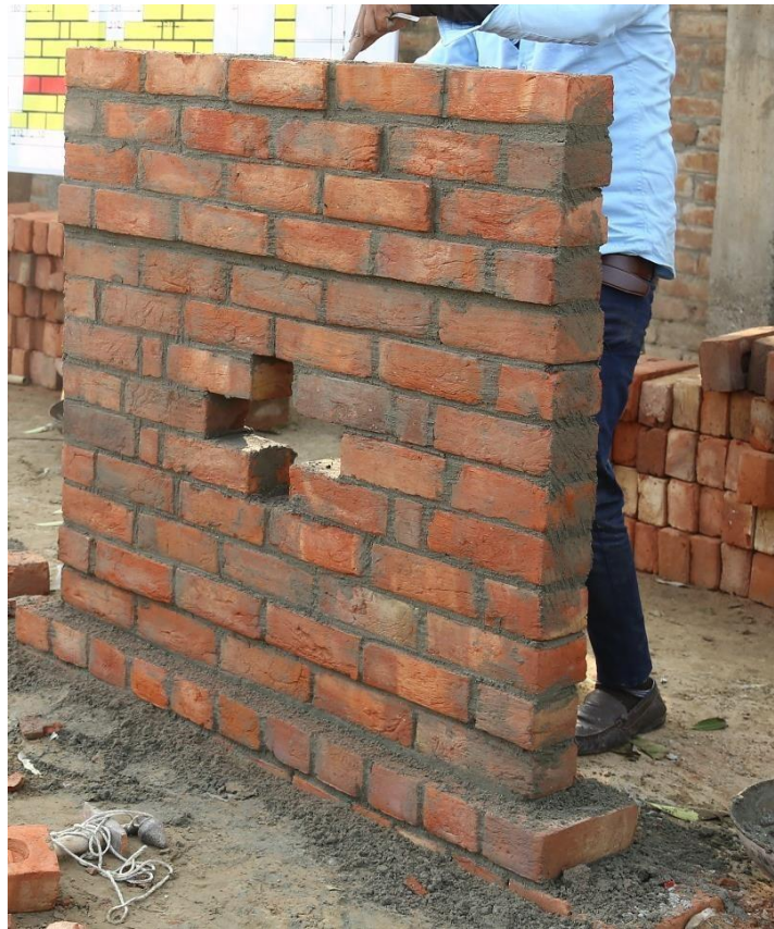
Construction of Wall Using Brickwork
