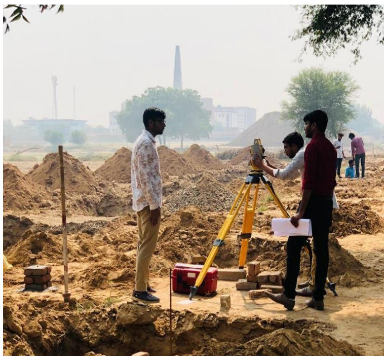
Surveying of Sewage Line in BFGI premises
