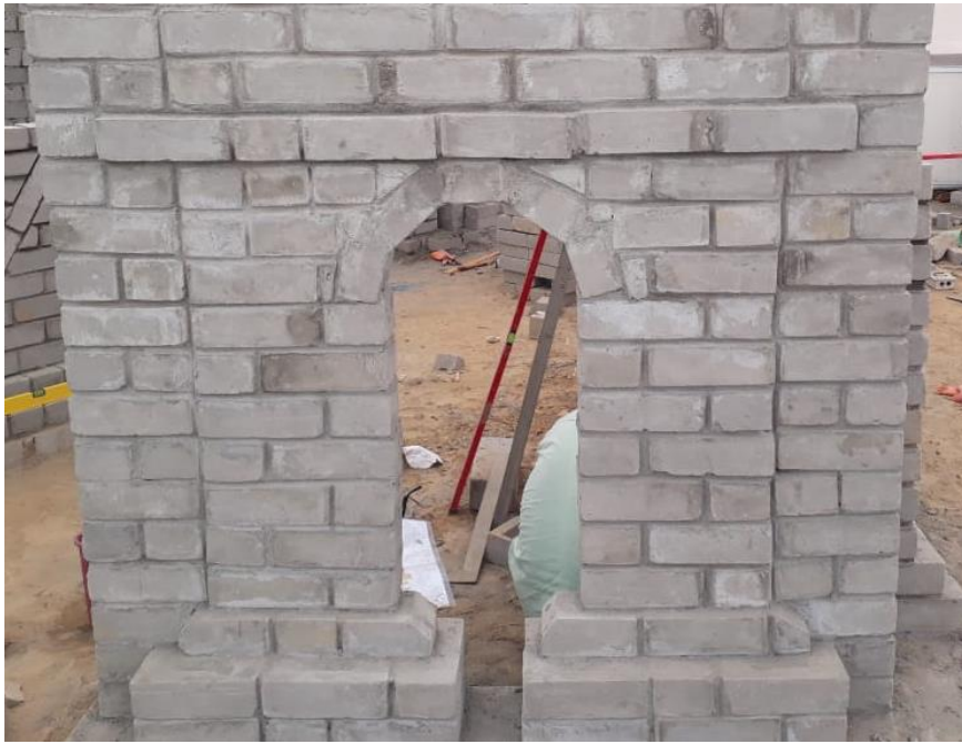
Project on Brick Laying task
