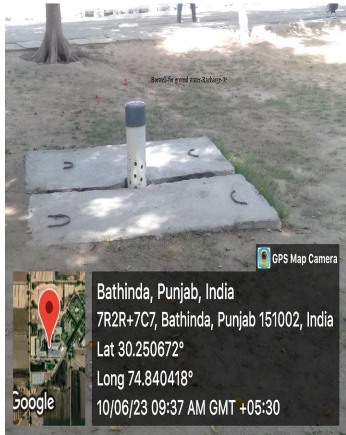
Figure 7: Water conservation (Water Recharging Point)
